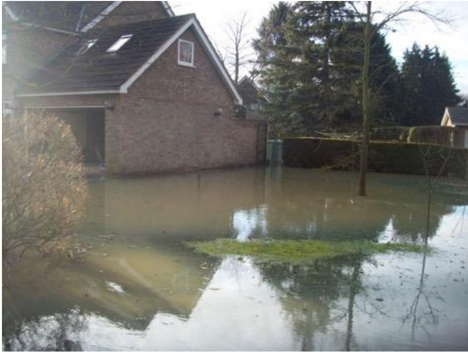
Flooding around a house & garage. 24Dec2020
