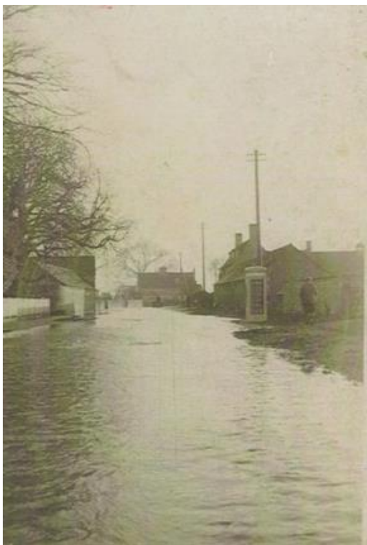
Greatford Main Street Flooding 27Aug1912
