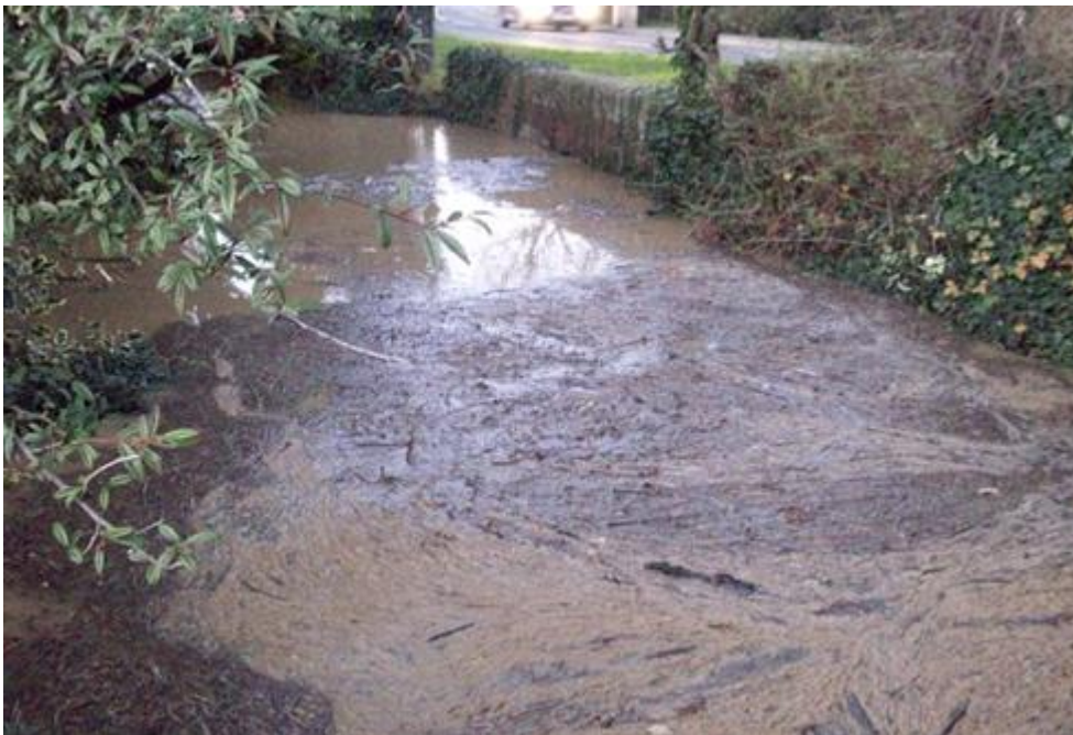
The junction of the small watercourse around Greatford Gardens with the drainage ditch alongside Carlby Road. The water is backing up against the brick front of the overloaded culvert under Carlby Rd (constructed 1837). The water height is above the flooded arch. Christmas 2020
